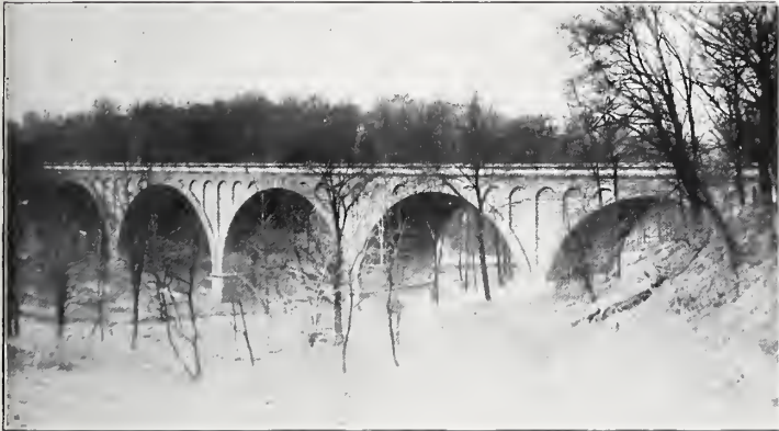
WASHINGTON PARK VIADUCT, CONCRETE
